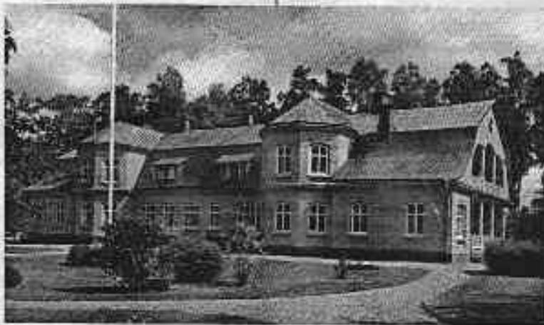
The Building housing the Eric Sahlström Institute, Tobo
